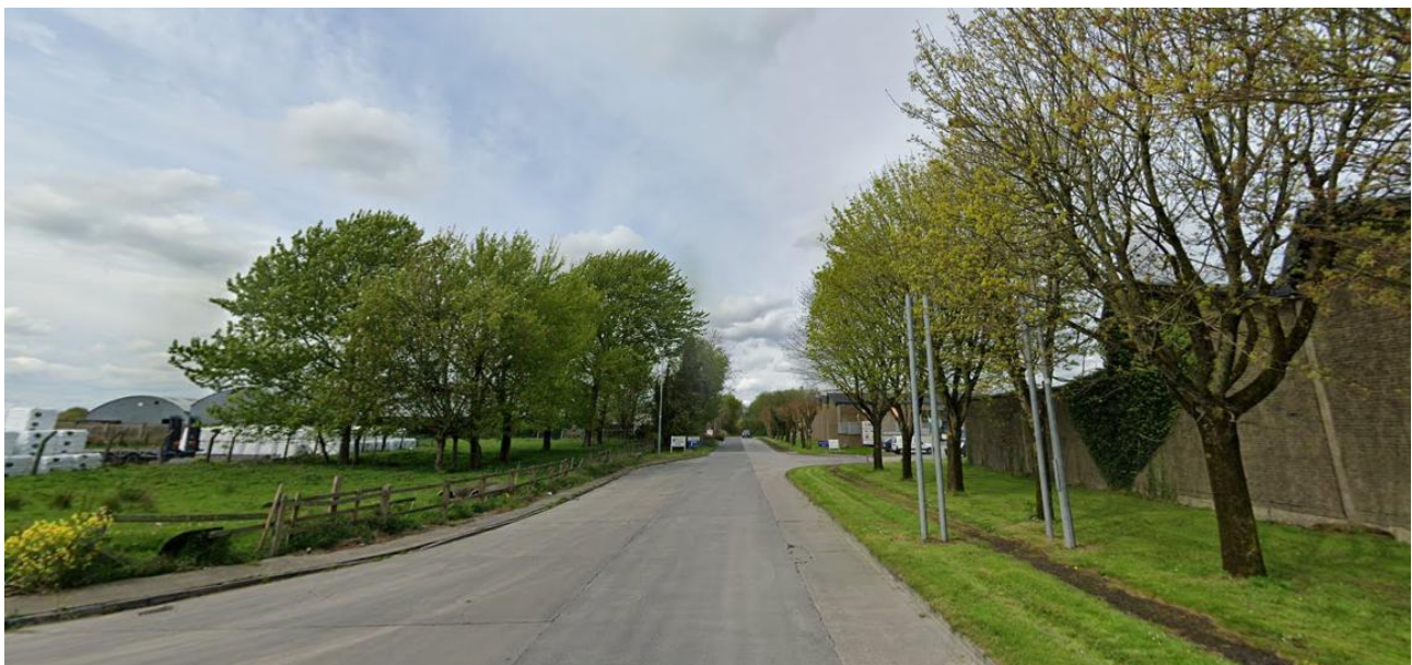
FIGURE 6-4: ACCESS ROAD TO CORCANREE BUSINESS PARK TO THE CORCANREE PUMP STATION SITE (SOURCE: GOOGLE MAPS)
