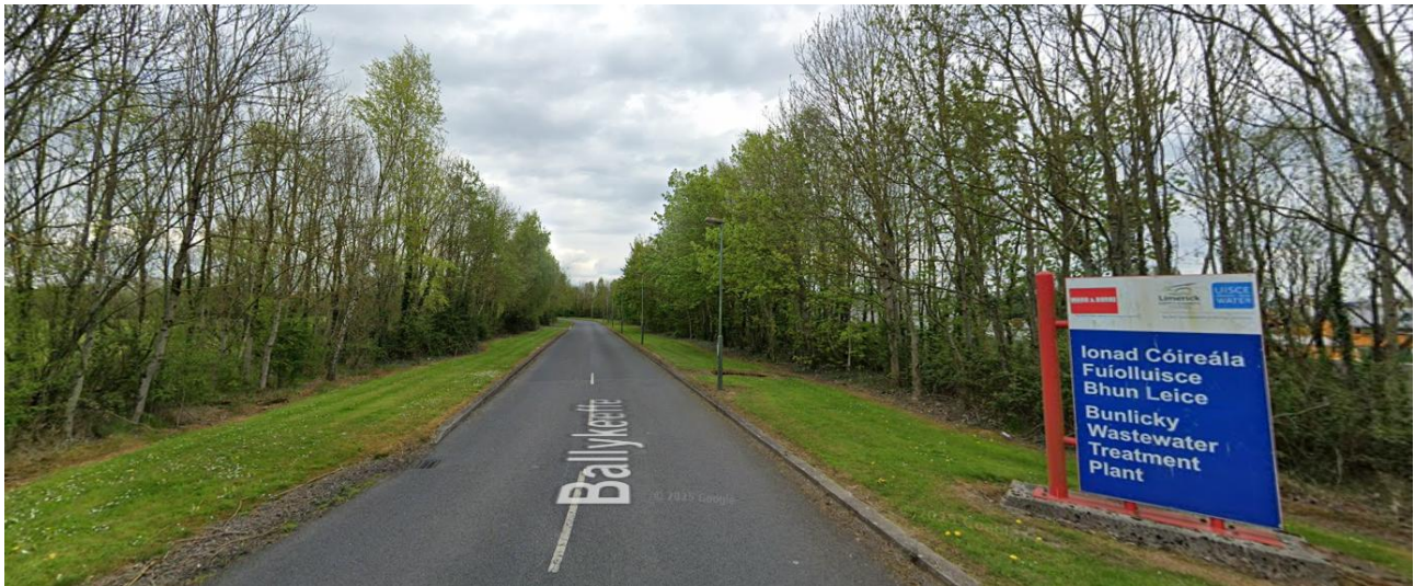
FIGURE 6-3: EXISTING LOCAL ACCESS ROAD TO THE LIMERICK WWTP SITE (SOURCE: GOOGLE MAPS)
